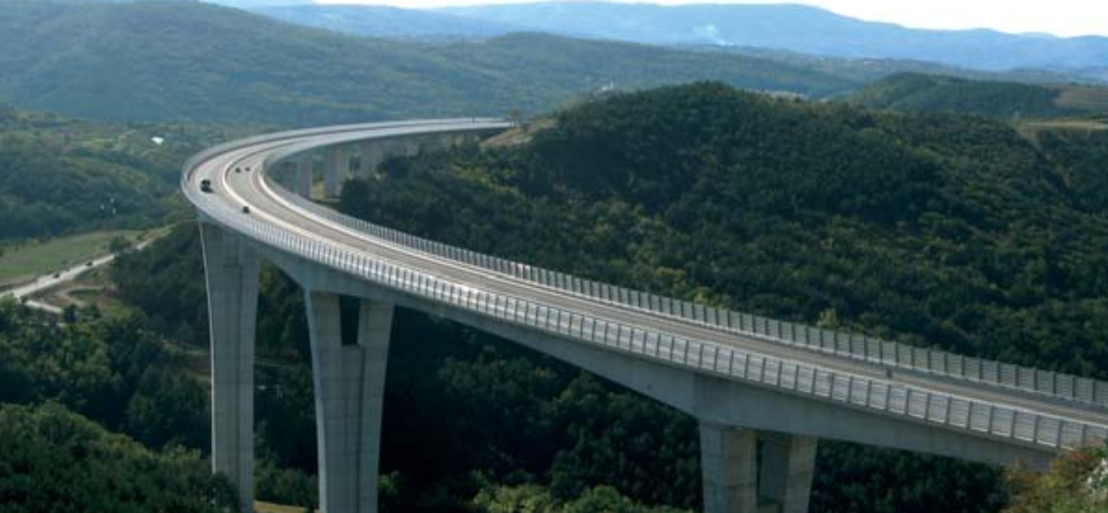
The new Črni Kal viaduct connecting central Slovenia with the Adriatic coast
